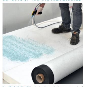
The **RENOLIT** DUALFIX adhesive is atomized onto the surface/insulation by means of a spray gun. The roofing membrane is being rolled and pressed onto the adhesive until sufficient initial bonding has taken place.
