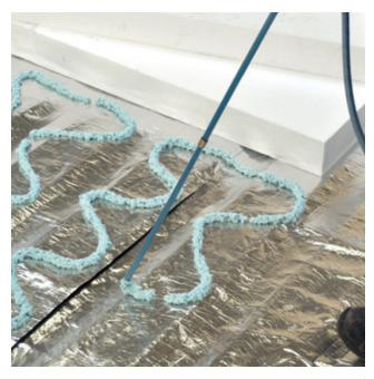
The RENOLIT DUALFIX adhesive is dispensed on the surface/insulation by means of a spray nozzle. The insulation panels are positioned and pressed onto the adhesive until sufficient initial bonding has taken place.
