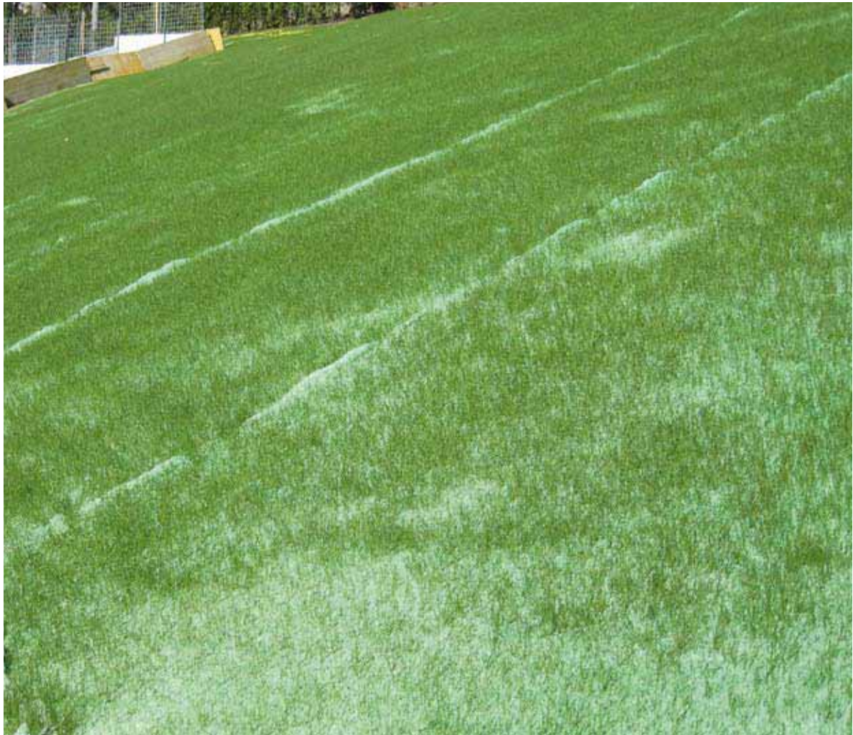
Initial stage of grass growing on a slope using KMat Mini L Sedum
