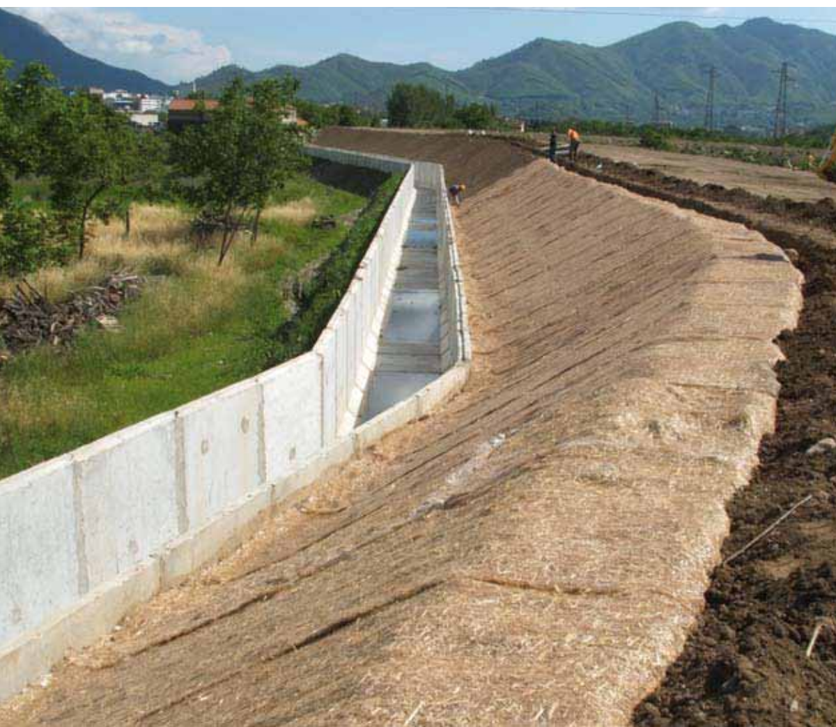
Ecologically sound reinforcement of the bank of a man-made canal using the Ecovermat anti-erosion mat
