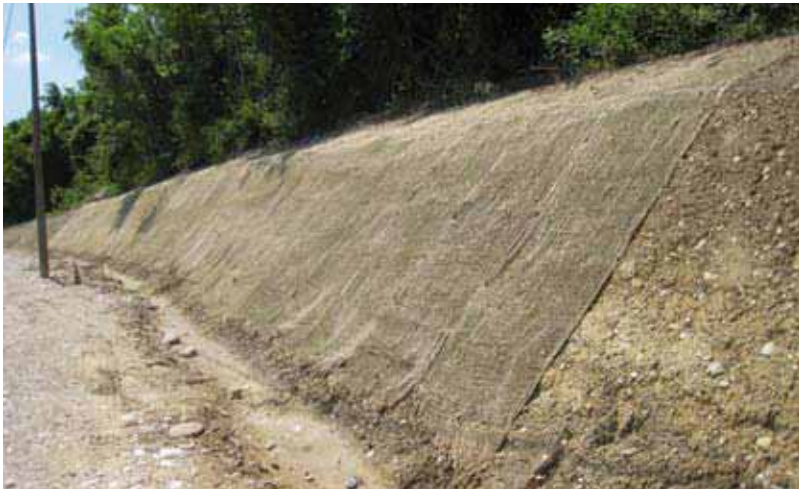
Installing Ecovernet J 500 in municipal road-works.
