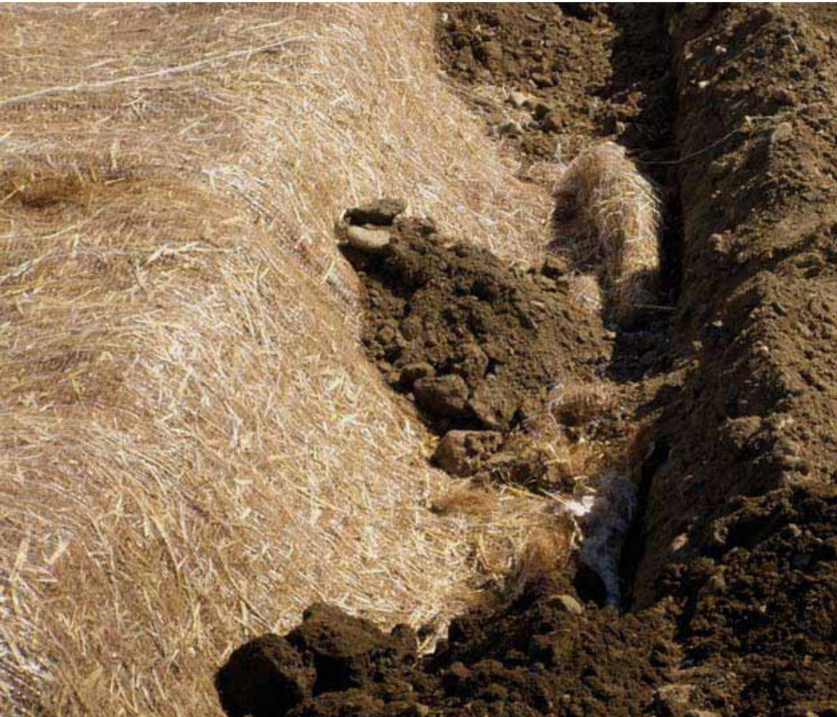
Detail of the biomat anchorage trench
