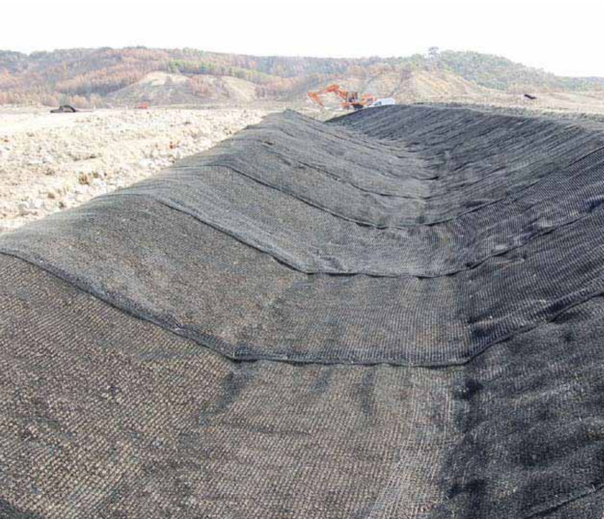
Lining a water course using a reinforced KMat RF 55 geomat
