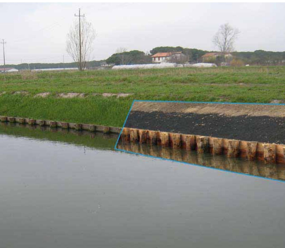
Anti-erosion stabilisation of a slope on the bank of a water canal using KMat L
