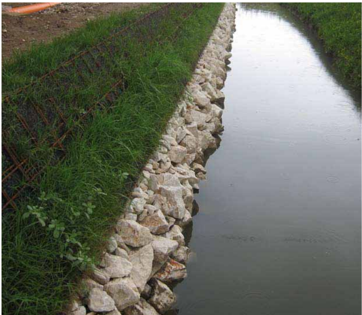
Building the bank of a water canal with Reinforced earthworks. The front-line anti-erosion component is KMat F Sedum.
