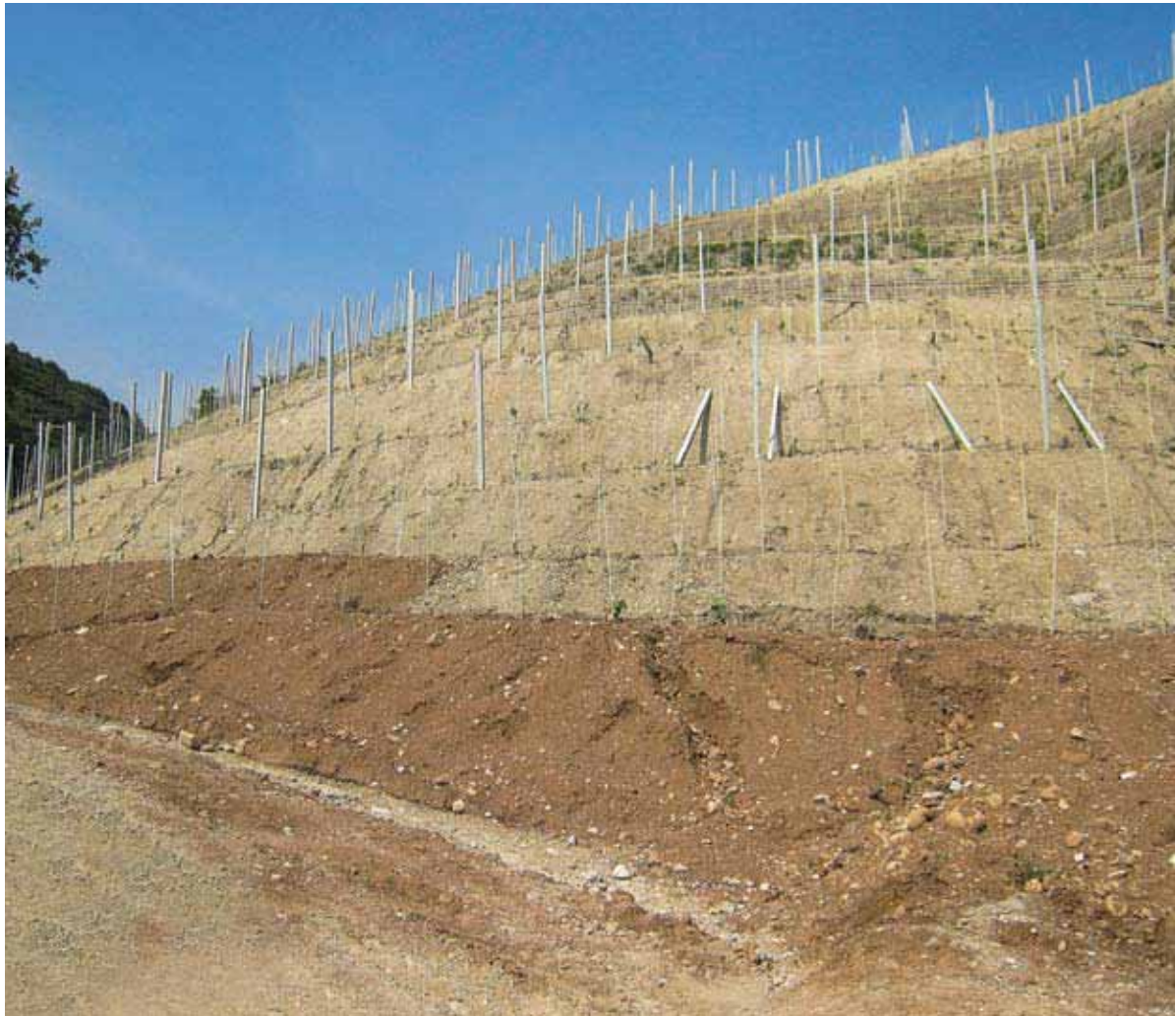
Use of XGrid to build a terraced vineyard
