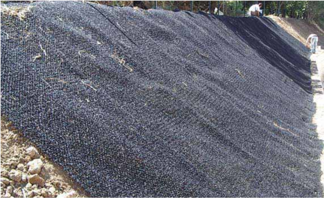
KMat used as the erosion control layer on a dry earth slope.
