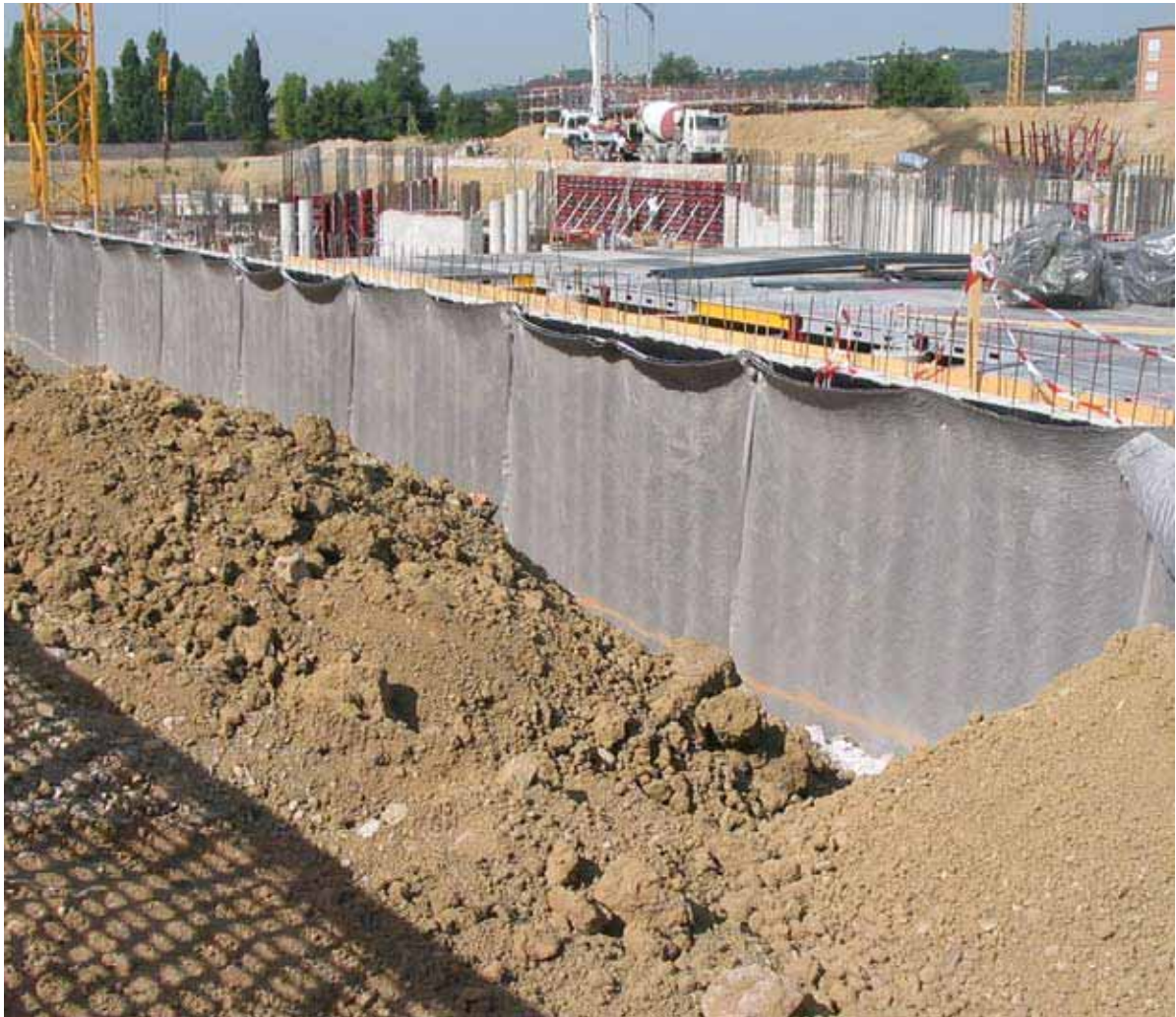
Protection of waterproofing and drainage in a shopping centre foundation
