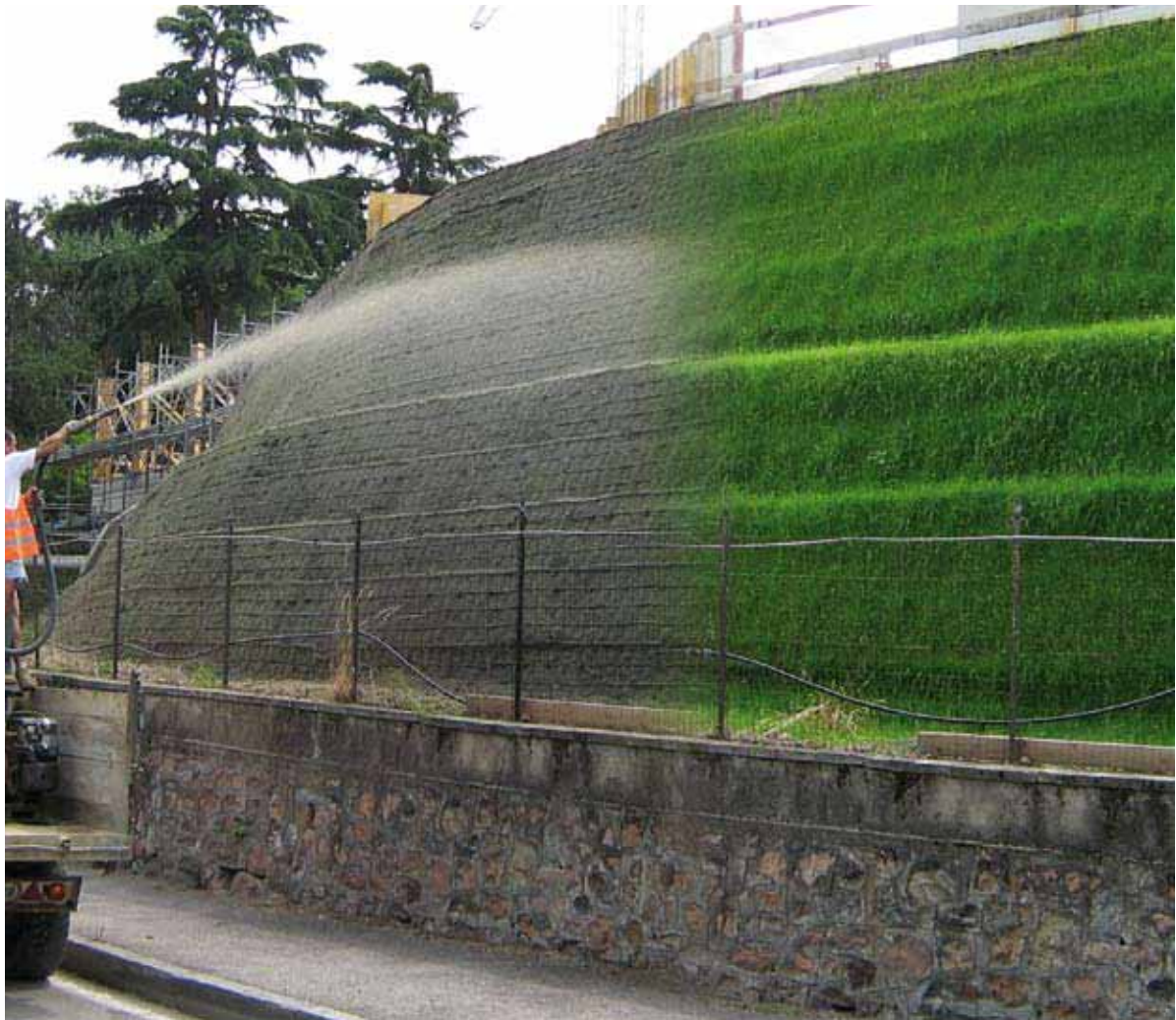
This photo montage shows the final stages of a Reinforced earthworks project: grass grown through hydroseeding and the result.
