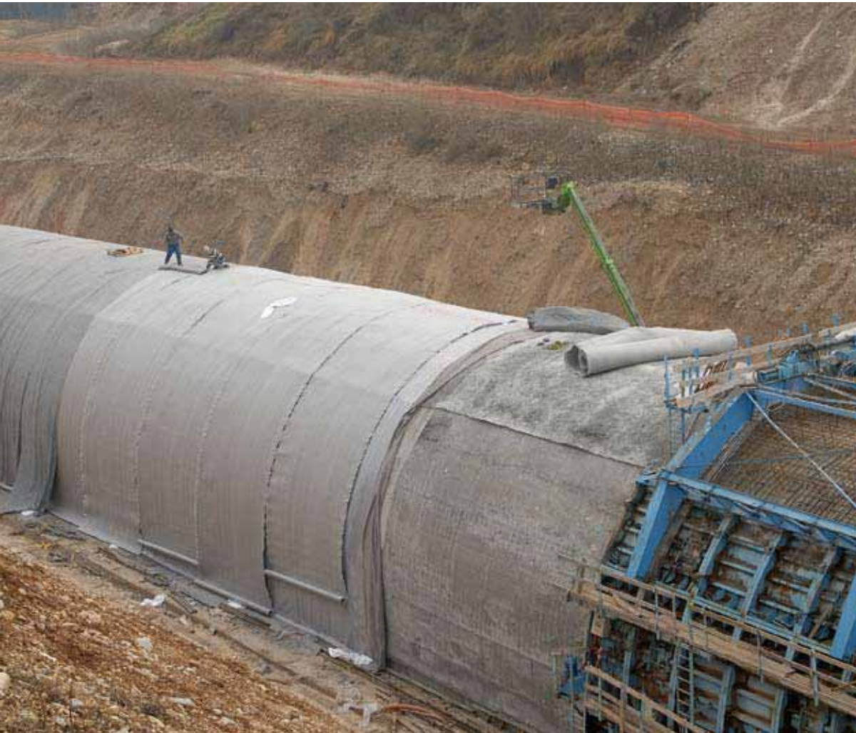
Extrados drainage of a man-made tunnel using QDrain C 20P
