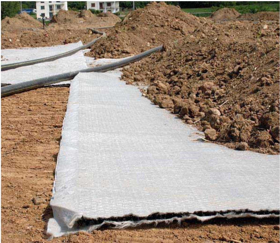
Landfill capping using QDrain ZW 8 14P
